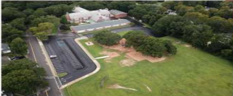
Ocean Ave ES Parking Lot Reconstruction
