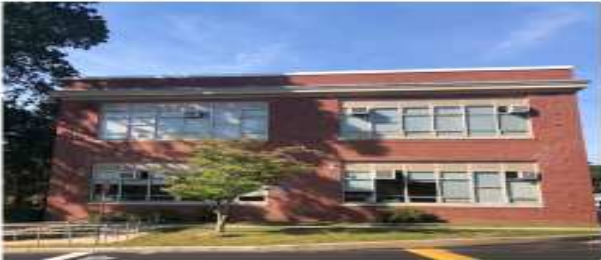
WJB Window Lintel Replacement and Brick Veneer Repair/Replacements
