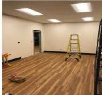
IT Room (old kitchen)
